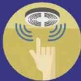
Test alarms at least once a month by pushing the test button.
